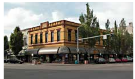
THE GRAY BUILDING 105-135 LIBERTY ST. NE - SALEM FULL BUILDING REMODEL
